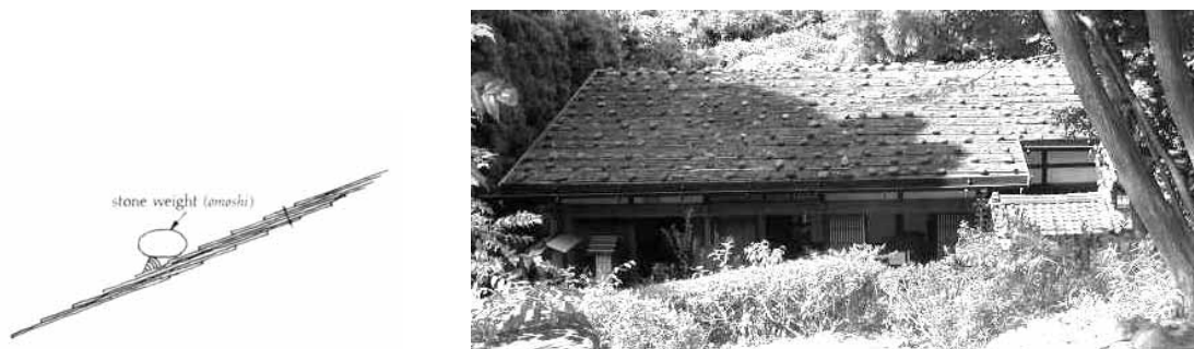
Fig. 12 – Plank roof held with stones 1
